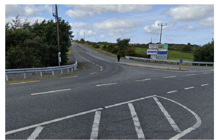
Image No. 9 (Looking Towards the Substation) Scale: NTS
